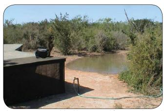
This permanent pit blind has a wood frame and wood walls to support the earth. The roof is plywood and the sides are a combination of nylon shade cloth and burlap. The front is left open for the photographer to cover with a combination of rough and fine mesh camo netting. Access is via a ramp and flap door in the back, or by crawling in the front.
